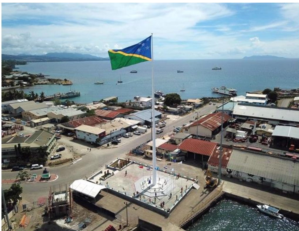
Figure 1: Point Cruz, Honiara. (Courtesy of the Solomon Islands Ports Authority)
